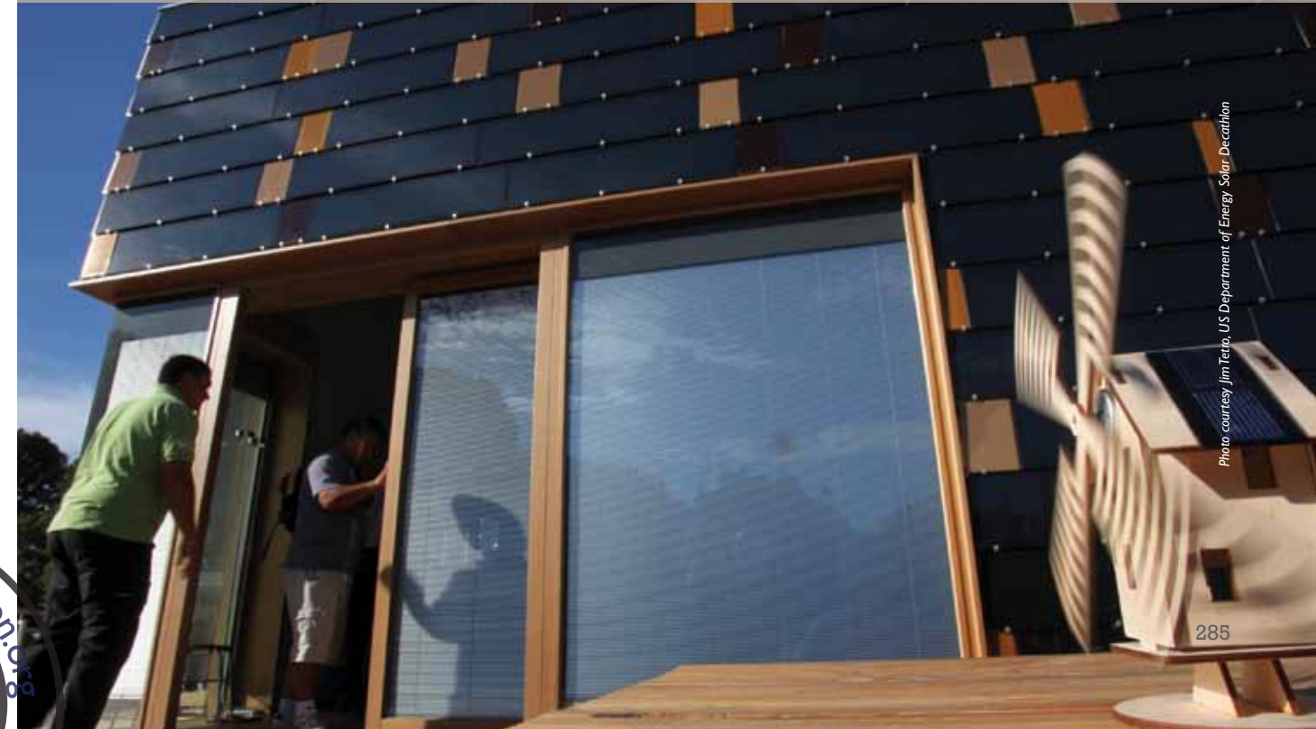
People take a first look inside the house of Technische Universität Darmstadt, Germany, on the opening day of the US Department of Energy Solar Decathlon 2009 in Washington, DC. Team Germany's house which integrated thin-film copper indium gallium selenide (CIGS) cells generates 200 percent of the house's energy needs and won overall first place.
